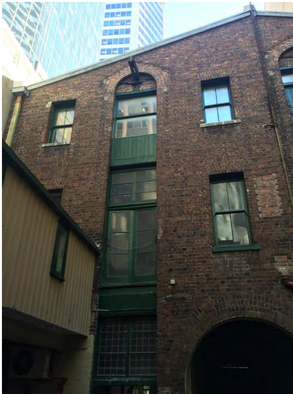
Figure 62 – Eastern elevation of warehouse. NBRSPartners, April 2015.
