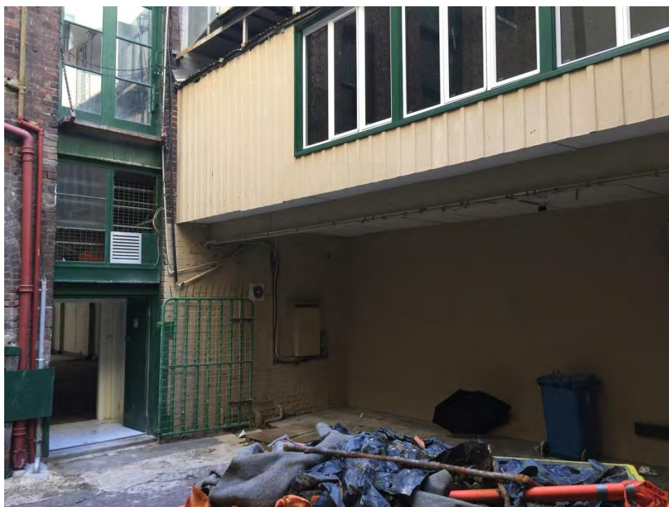
Figure 78 – Yard (Y02) looking southeast. NBRSPartners, April 2015.
