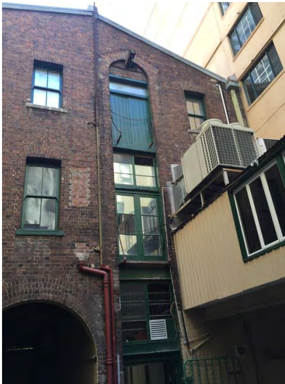
Figure 59 – Eastern elevation of warehouse. NBRSPartners, April 2015.
