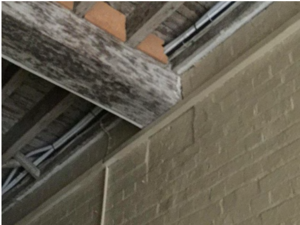
Figure 73 – Timber beam borne on stone block in wall of Cartway (Y01) NBRS+Partners, April 2015.
