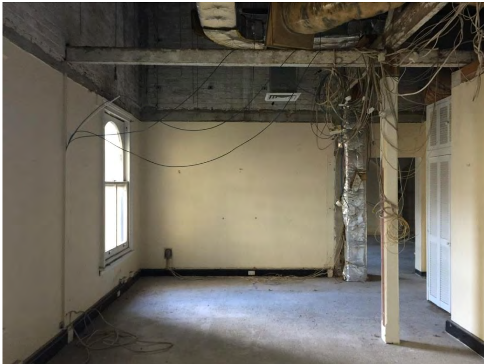
Figure 93 – Western section of space S02 showing timber post, beam and truss structure. NBRSPartners, April 2015.
