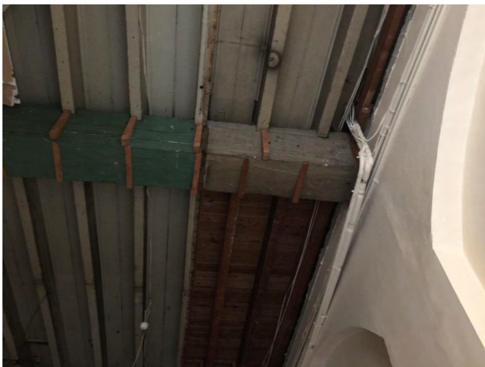
Figure 91 – South-western corner of space G06 showing original matchboard lining. NBRSPartners, April 2015.
