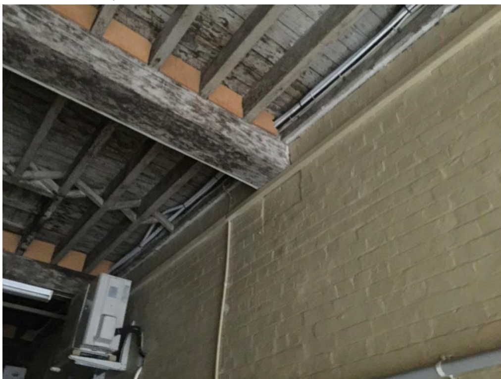
Figure 72 – Timber beam borne on stone block in wall of Cartway (Y01) NBRS+Partners, April 2015.
