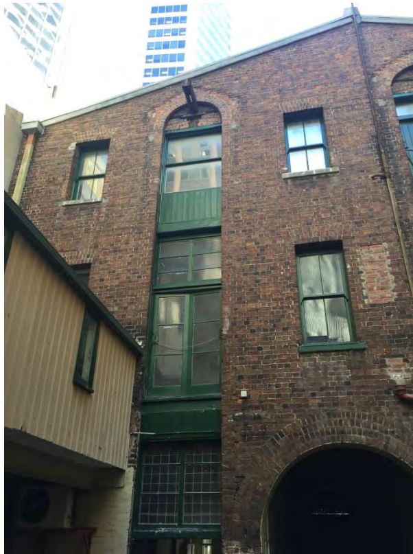
Figure 61 – Eastern elevation of warehouse. NBRSPartners, April 2015.
