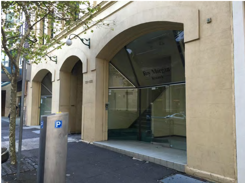
Figure 49 – Ground floor on Sussex Street. NBRSPartners, April 2015.
