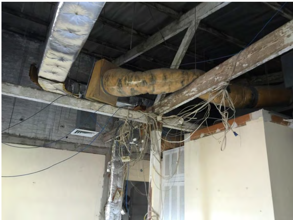
Figure 94 – Western section of space S02 showing timber post, beam and truss structure. Recent studwork walls to stair and service core at right. NBRSPartners, April 2015.
