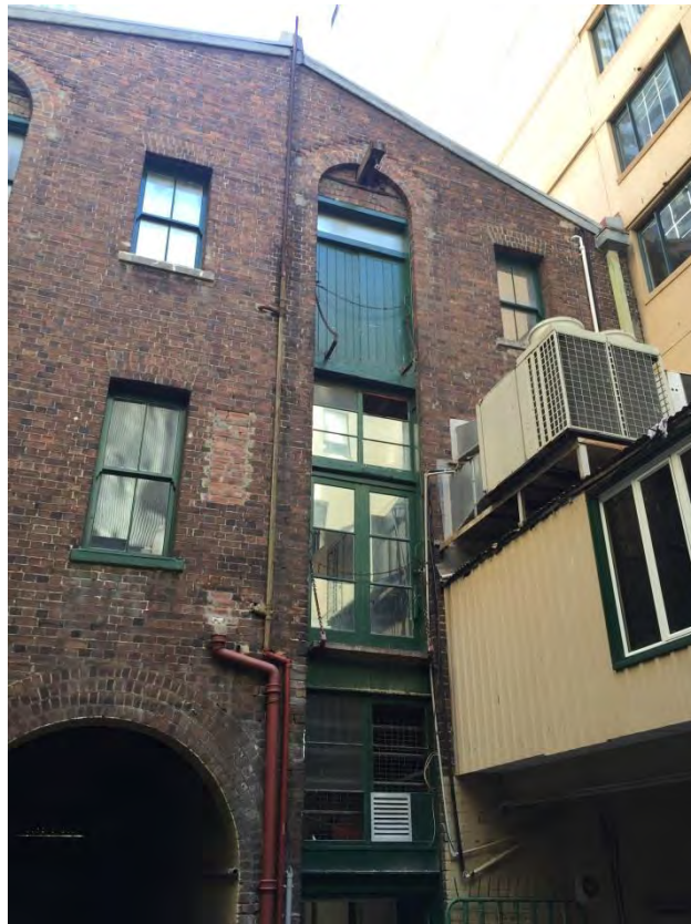
Figure 63 – Eastern elevation of warehouse. NBRSPartners, April 2015.
