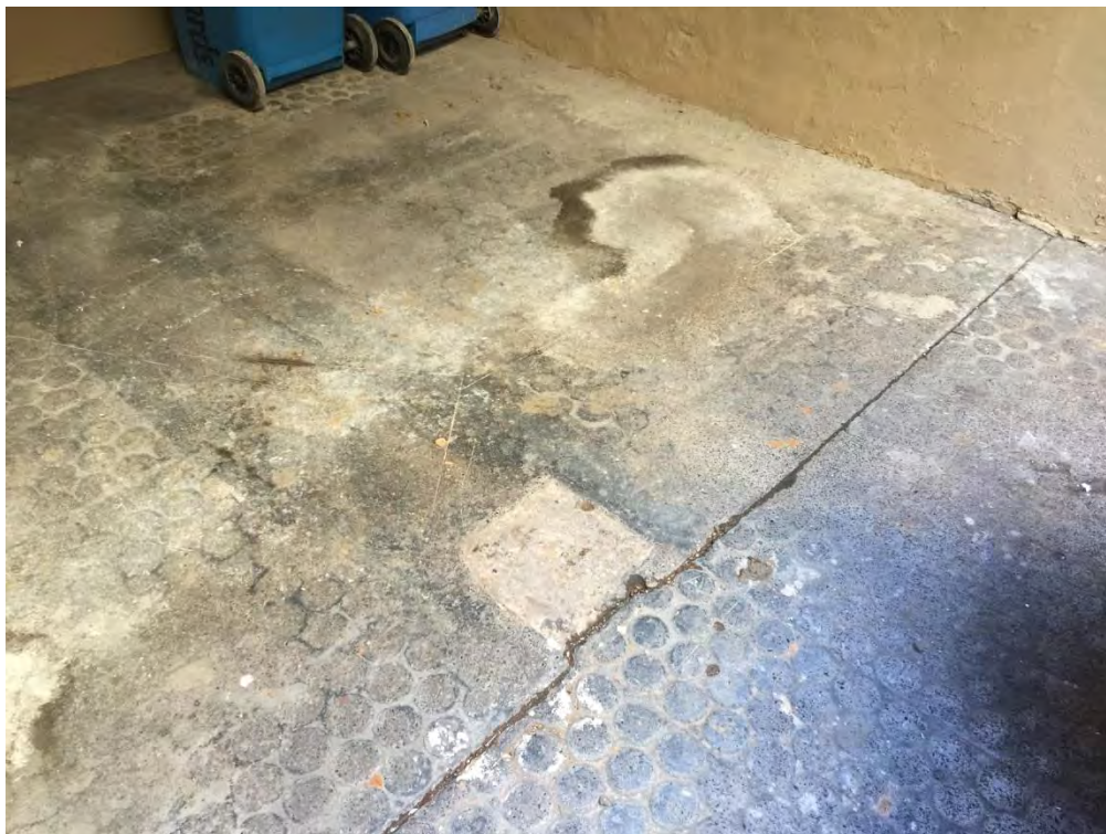
Figure 80 – One of five sandstone block footings for posts evident in floor of yard (Y02). NBRSPartners, April 2015.
