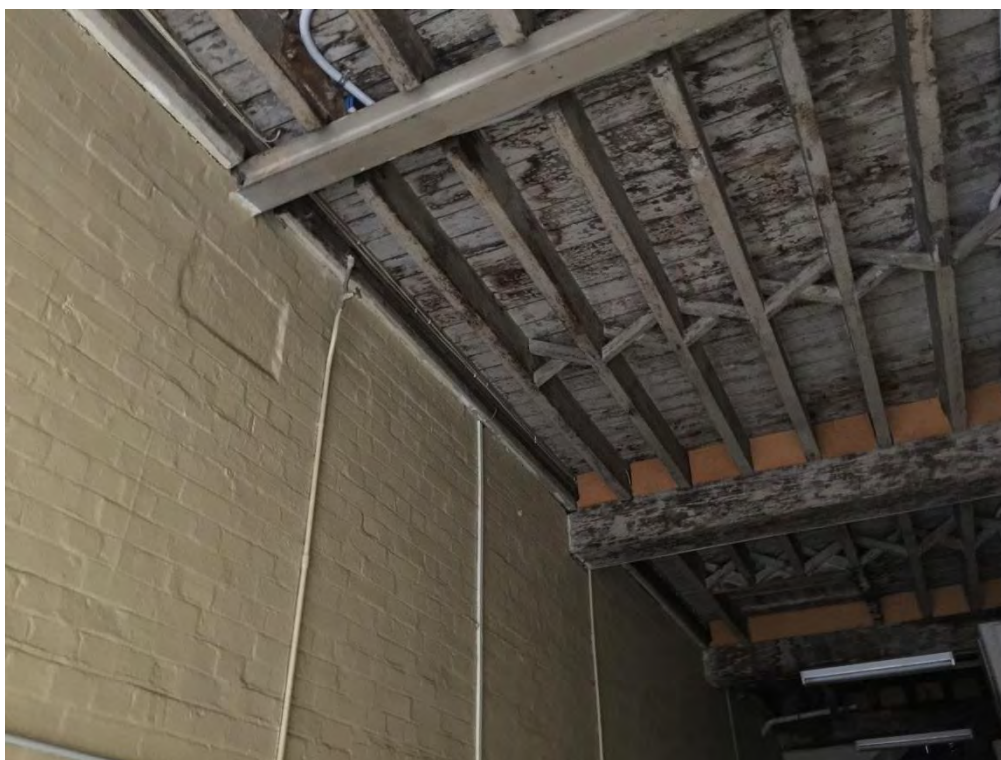
Figure 71 – Steel beam in place of timber beam borne in wall of Cartway (Y01) NBRS+Partners, April 2015.
