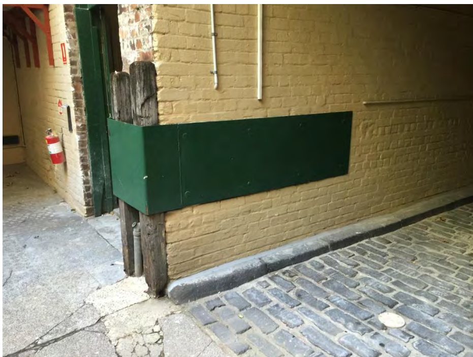
Figure 68 – Timber guard posts and steel guardrail at eastern entrance to cartway (Y01) showing recent granolithic paving of yard (Y02) and stone setts and curbs of cartway.. NBRSPartners, April 2015.
