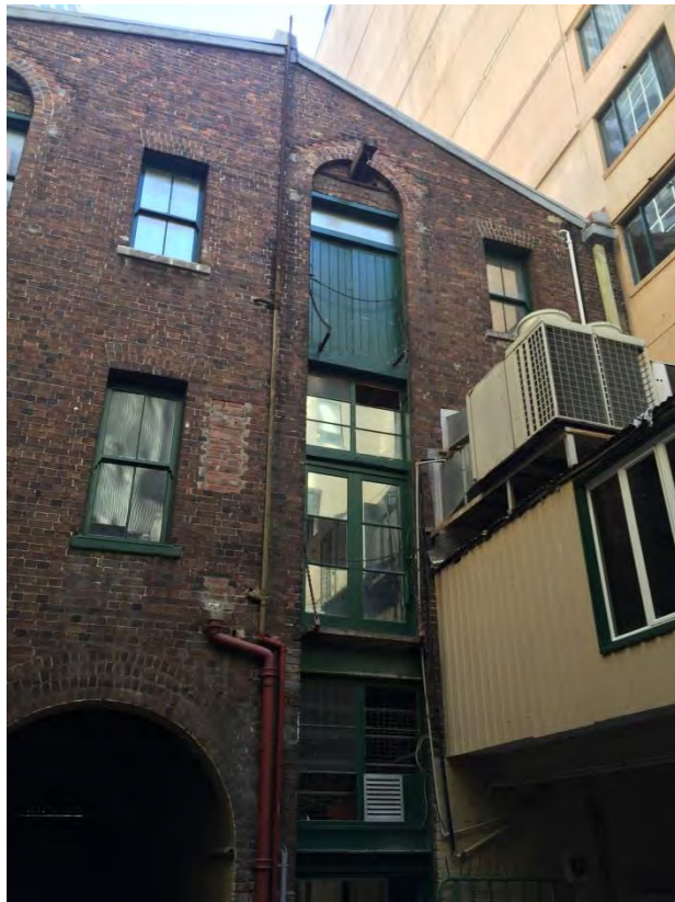
Figure 64 – Eastern elevation of warehouse. NBRSPartners, April 2015.
